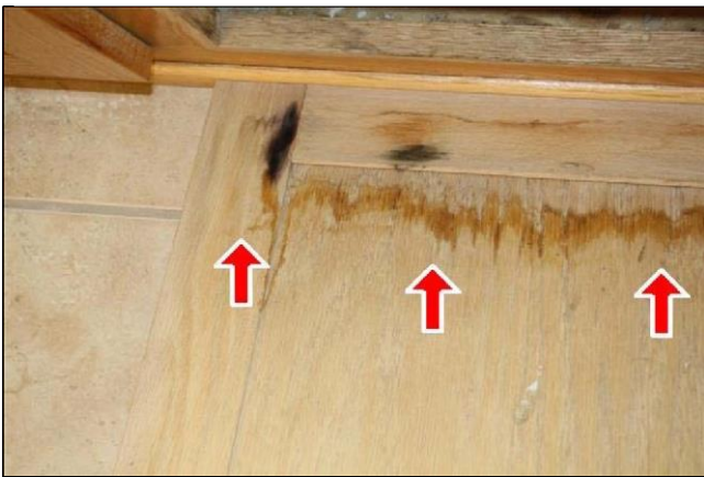
9.4 Item 3(Picture) Black staining, water stains on tub access panel
