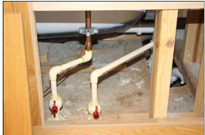
9.4 Item 2(Picture) Tub access area
