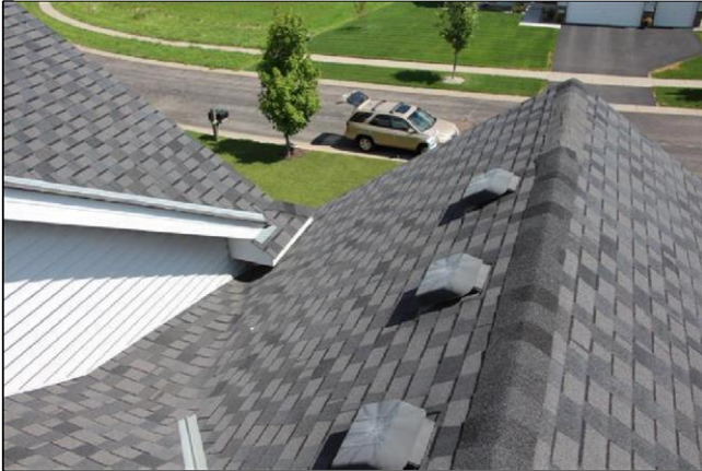
1.0 Item 3(Picture) Above Garage Roof
