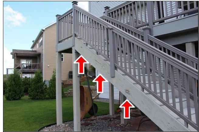
2.5 Item 2(Picture) Deck stringer paint failing
