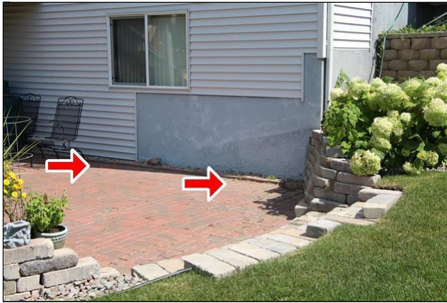
2.8 Item 1(Picture) Drainage concern--brick border
