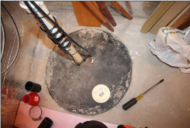
5.6 Item 1(Picture) Sealed sump pump cover
