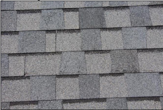
1.0 Item 1(Picture) Roof Condition
