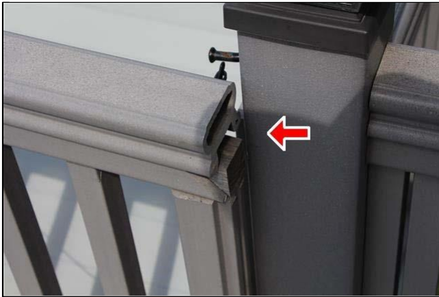
2.5 Item 1(Picture) Railing gate won't close
