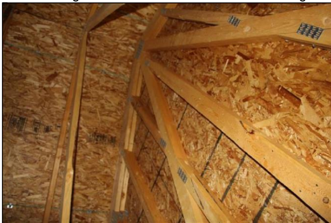
1.4 Item 1(Picture) Attic End Wall
