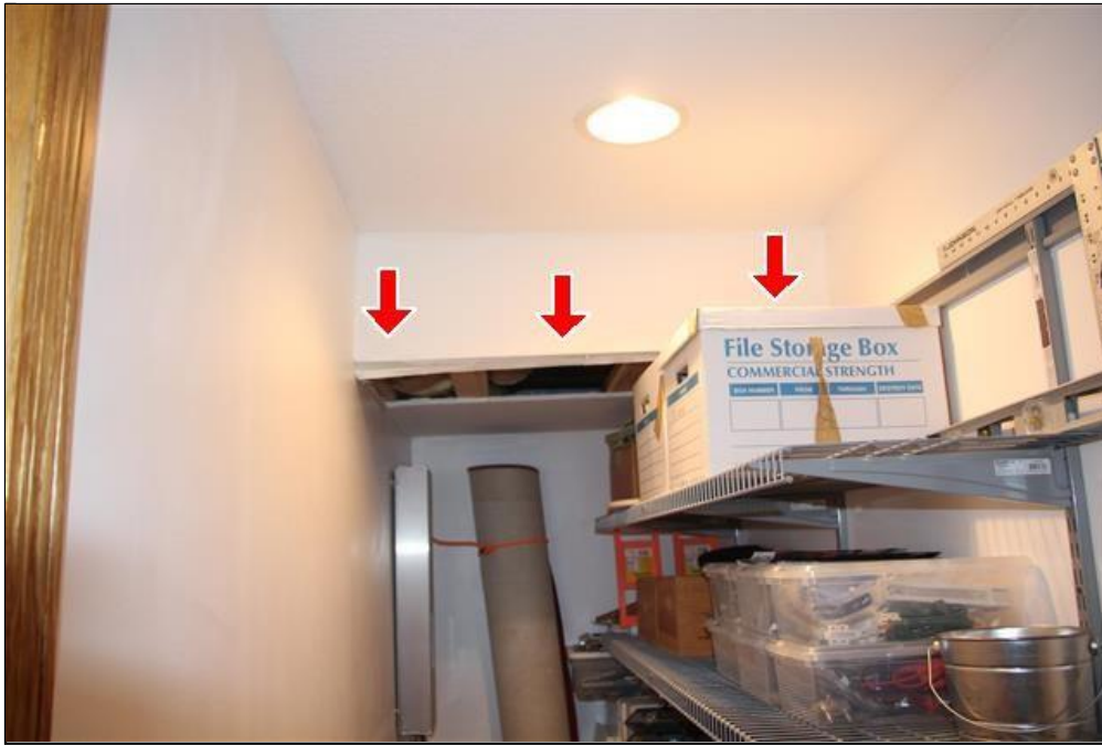
9.0 Item 2(Picture) Water staining on drywall
