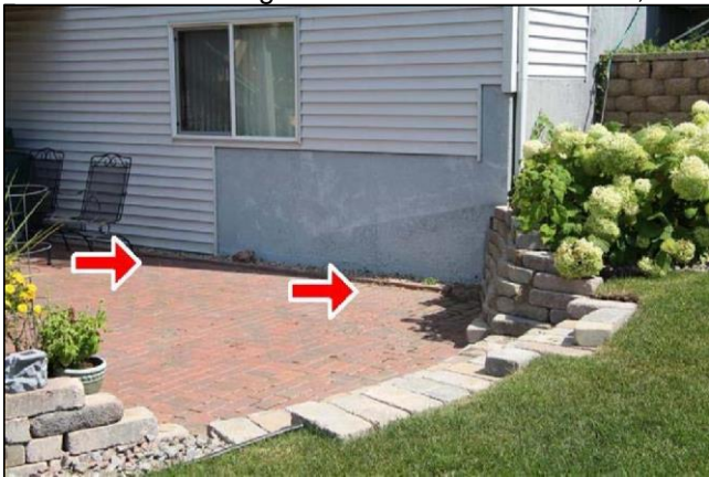
2.8 Item 1(Picture) Drainage concern--brick border
