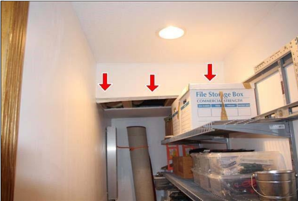
9.0 Item 2(Picture) Water staining on drywall
