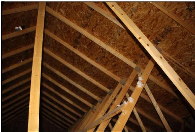
1.4 Item 3(Picture) Attic along ridge
