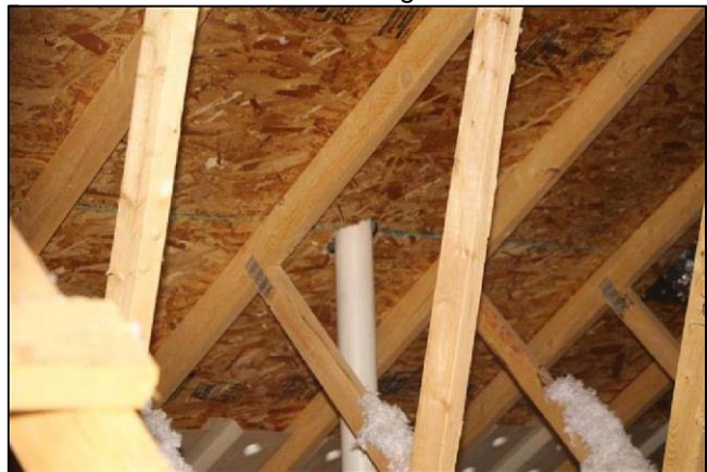
1.4 Item 2(Picture) Attic Framing Structure
