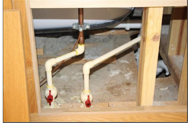
9.4 Item 2(Picture) Tub access area
