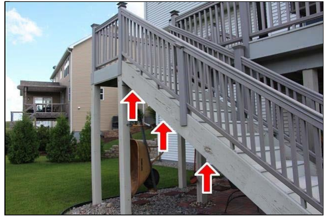
2.5 Item 2(Picture) Deck stringer paint failing
