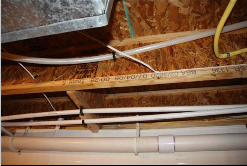
3.4 Item 1(Picture) Floor Joists
