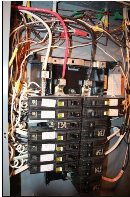
6.2 Item 2(Picture) Distribution Panel
