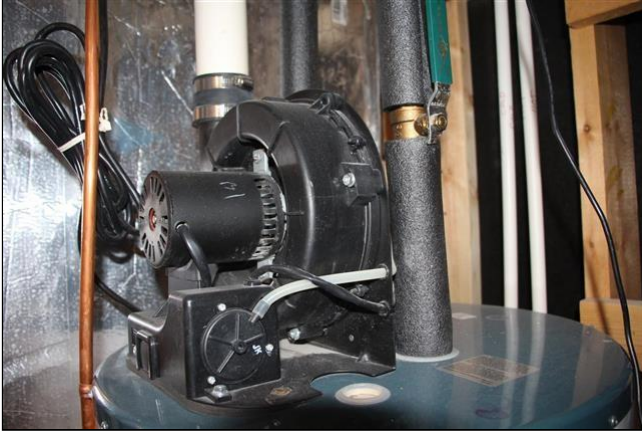
5.2 Item 1(Picture) Water Heater Venting uses mechanical assist
