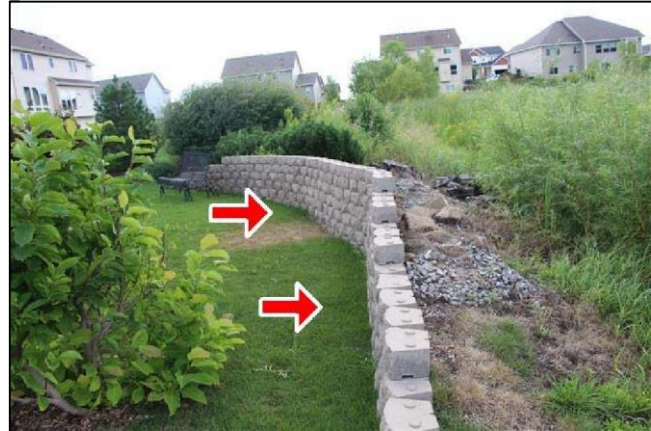
2.8 Item 4(Picture) Backyard keystone block wall used to retain dirt
