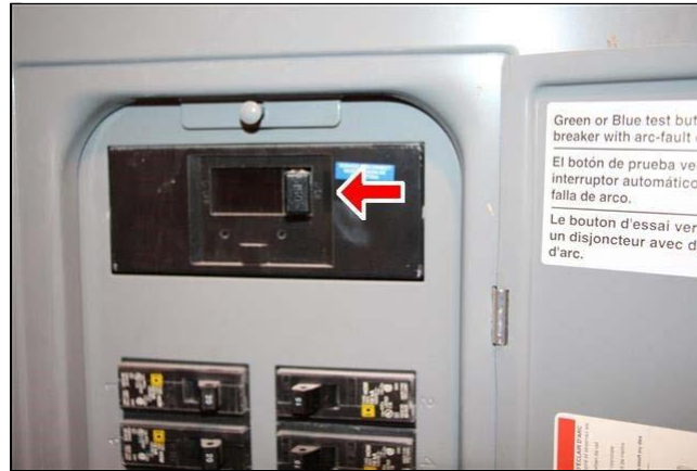
6.6 Item 2(Picture) 150 Amp service panel
