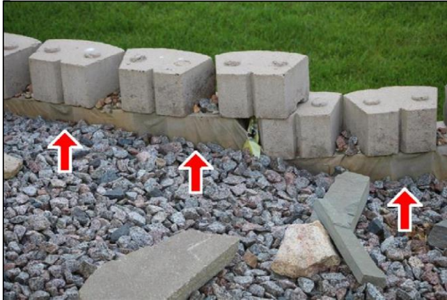
2.8 Item 3(Picture) Drainage diverted around block
