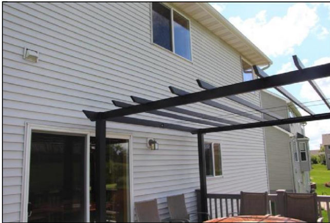
2.4 Item 2(Picture) Above Deck Shade Structure
