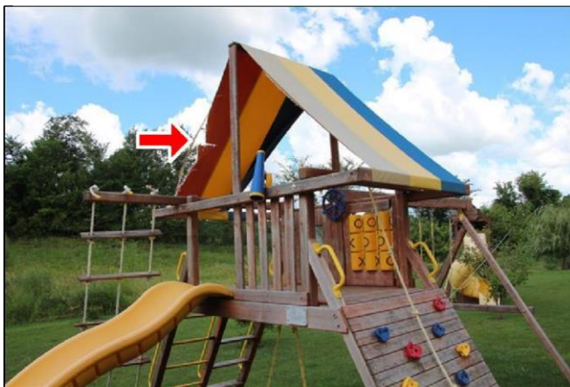
2.4 Item 4(Picture) Back yard play structure--Canopy torn
