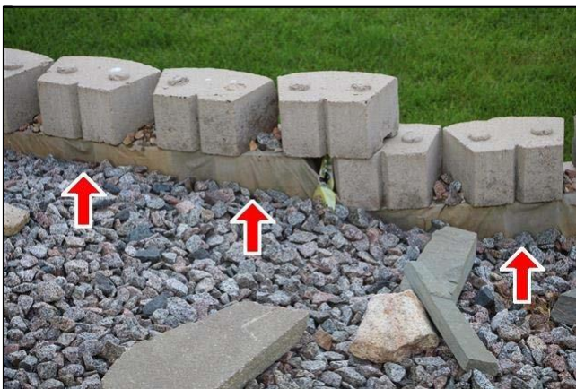
2.8 Item 3(Picture) Drainage diverted around block
