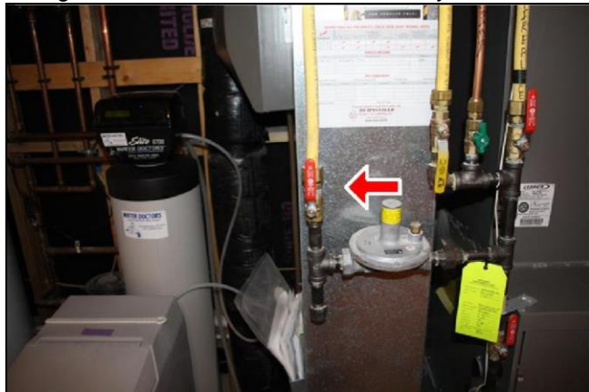
5.1 Item 1(Picture) Gas shut-off valve
