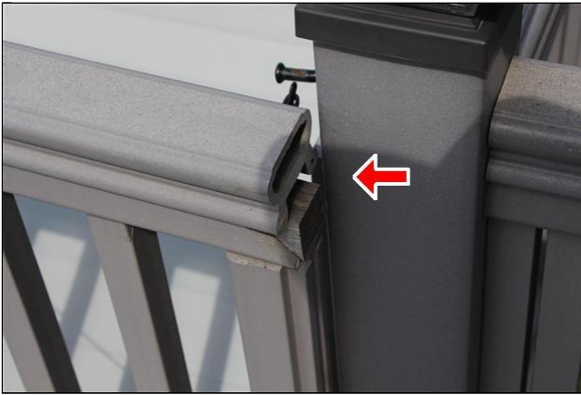
2.5 Item 1(Picture) Railing gate won't close
