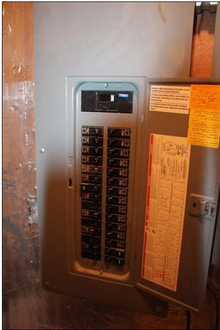
6.6 Item 1(Picture) Main panel
