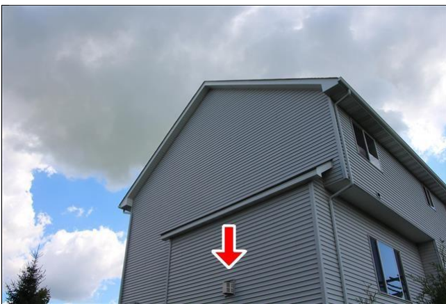
7.2 Item 1(Picture) Fireplace flue through wall
