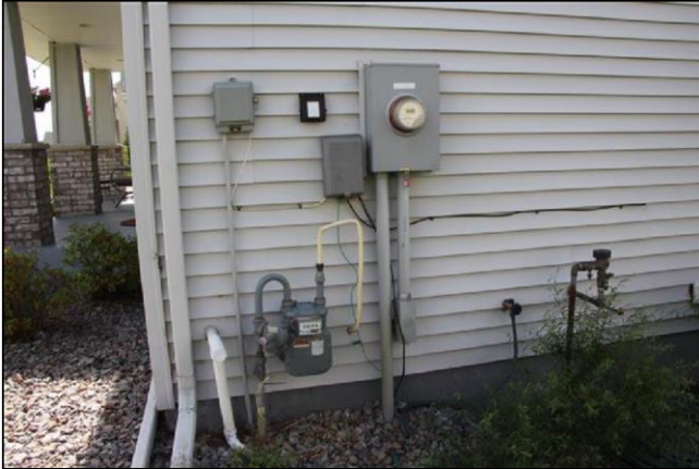
6.0 Item 1(Picture) Service Entrance
