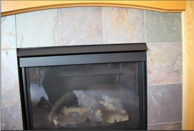
7.0 Item 1(Picture) Gas Fireplace
