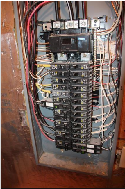
6.2 Item 1(Picture) Main Panel
