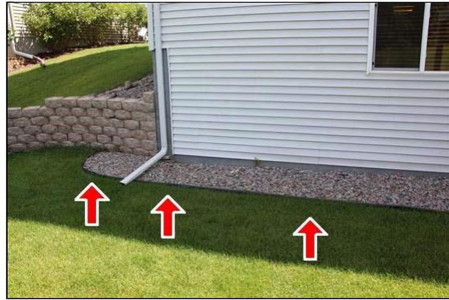
2.8 Item 2(Picture) Drainage concern--rubber border
