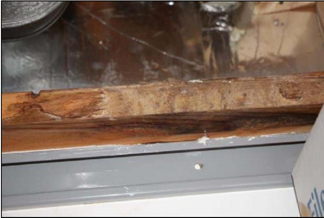
9.0 Item 1(Picture) Water staining & discoloration on ceiling framing.
