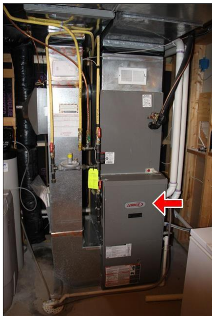
4.0 Item 1(Picture) Lennox Heating & Cooling System
