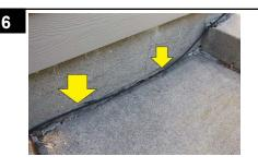
LOCATION: Exterior SYSTEM: ExteriorCONDITION: There is cracking between the walkway and the foundation.EXPLANATION: Water that can penetrate below grade along the foundation can seep into the basement.
