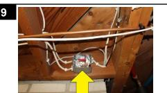
LOCATION: Basement SYSTEM: Electrical CONDITION: Exterior junction box cover plate is missing by chimney
