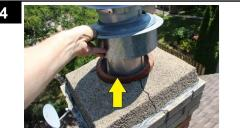
**LOCATION:** Chimney - Metal **SYSTEM:** Roof **CONDITION:** The flue collar is loose
