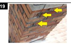
LOCATION: Chimney - Masonry SYSTEM: Roof CONDITION: Chimney masonry is deteriorated EXPLANATION: Deterioration of chimney brick masonry is observed. IMPACT/CONSEQUENCES: Brick masonry serves to support, enclose, and provide weatherproof protection of chimney flues. Brick masonry that is deteriorated will not meet its intended functions. Further and ongoing deterioration may result in costly repairs, and in some circumstances can be a safety concern. Repair by a masonry specialist is recommended.
