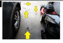
LOCATION: Garage FloorSYSTEM: ExteriorCONDITION: Garage concrete floor displays pitting (minor)EXPLANATION: The concrete is pitted. The cause may be due to moisture and/or<br/>corrosive chemicals. There are companies that apply acceptable sealers on the<br/>concrete to slow or prevent this condition.
