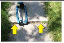
LOCATION: Exterior Rear SYSTEM: Exterior CONDITION: Walking surface has settled or heaved
