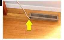
**CONDITION:** Non-conforming wiring observed **EXPLANATION:** Wiring is observed to be done in a manner that does not appear to be in accordance to current standards. The cable wire is running through the supply register.
